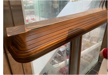
Above: Installation of handrail on site. down: Fabrication of the cast stainless steel posts.
