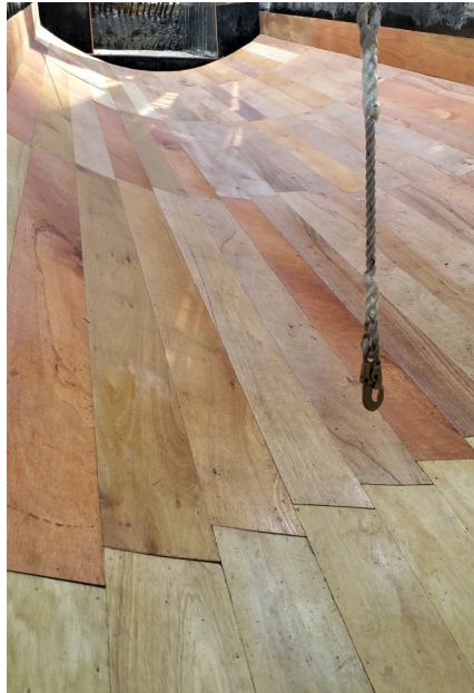
Timber formwork and metal mesh.
