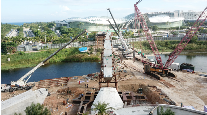
Photograph of construction site
