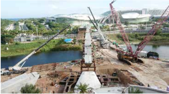
Photograph of construction site
