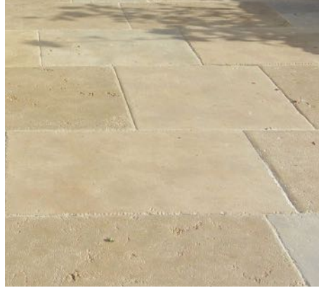
Paving in local limestone
